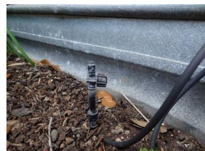
Micro sprayers are available with valves so water can be turned off at any given emitter when not needed.
